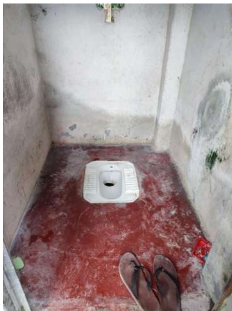
Toilet of Sheikh Sohrab Ali, Datinakhali
