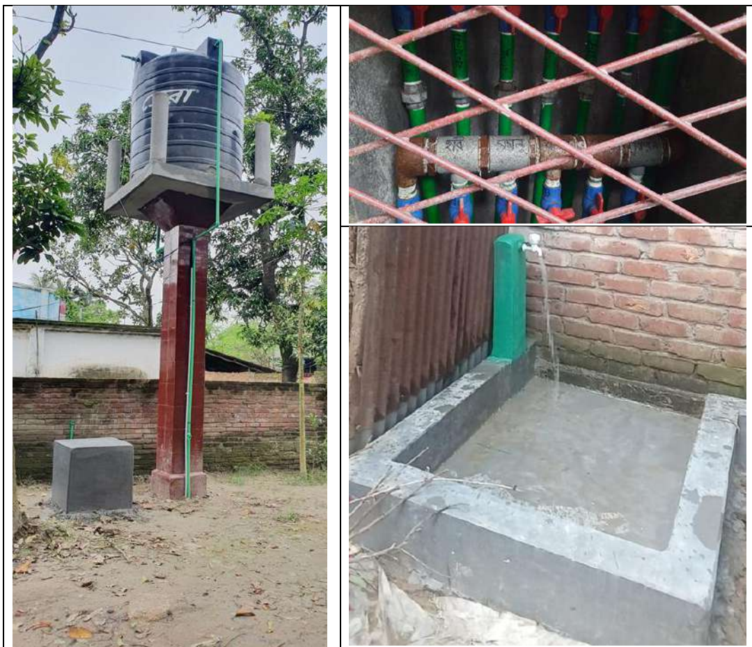
Figure 5.2: Mini Piped Water Supply System
