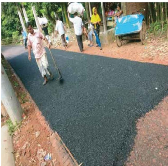
Waste plastic and asphalt are being laid on the base course
