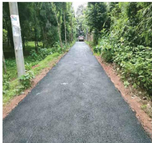
Asphalt Pavement with Waste Plastic
