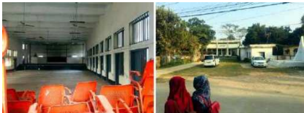
Figure 7.8: Existing Condition of Upazila Auditorium
