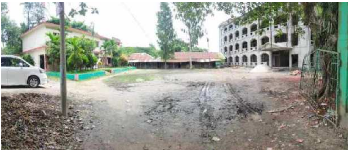
Figure 7.20: Existing Condition of Saikchail Government Primary School, Monohorgonj
