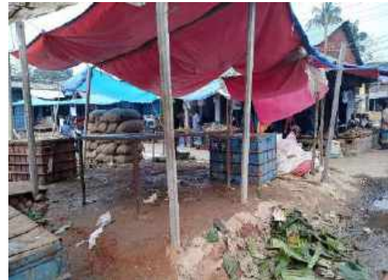
Fig: vulnerable structure
