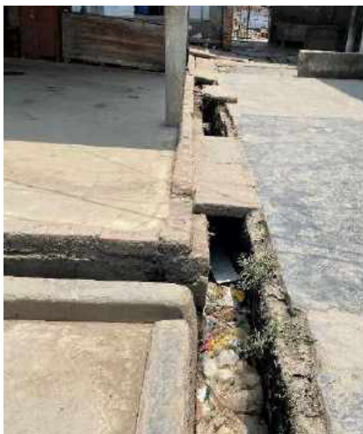
Fig: drainage system in existing bazaars
