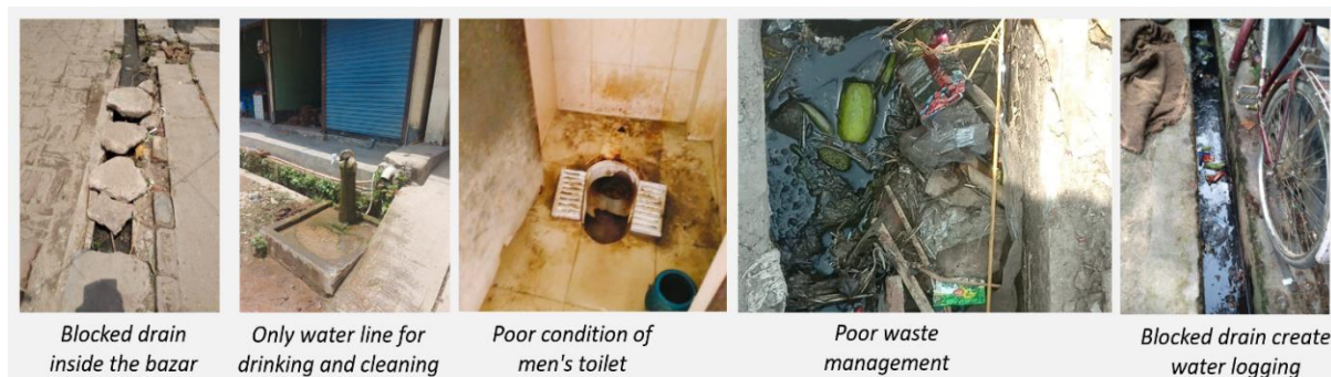
Figure 6-9: Current status of infrastructure
