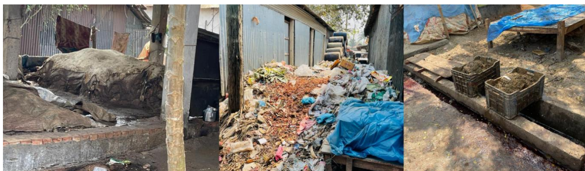
Poor market facility at Chalakchar market
