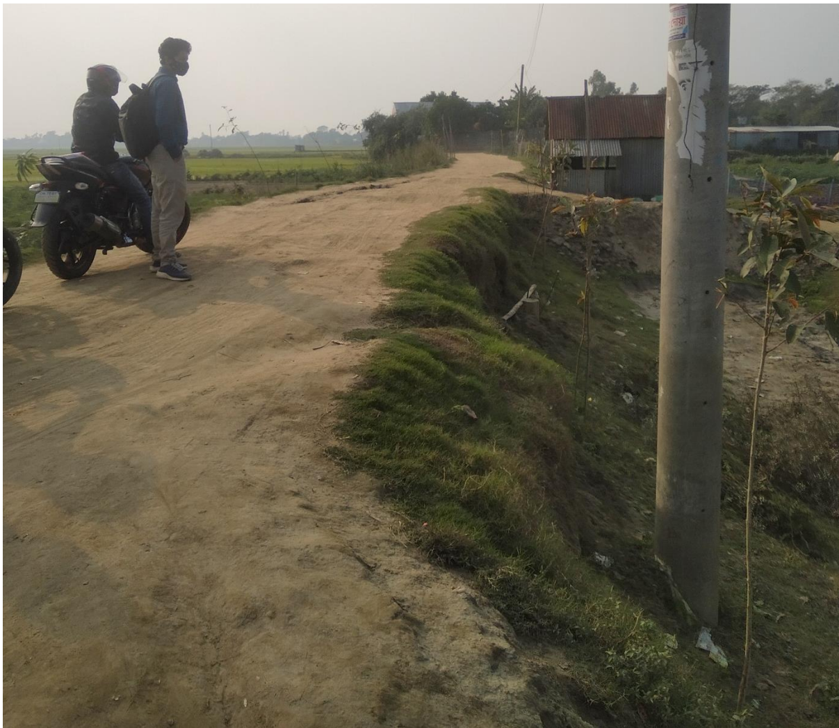
Figure 9: Condition of the visited road alignment at Case Study union
