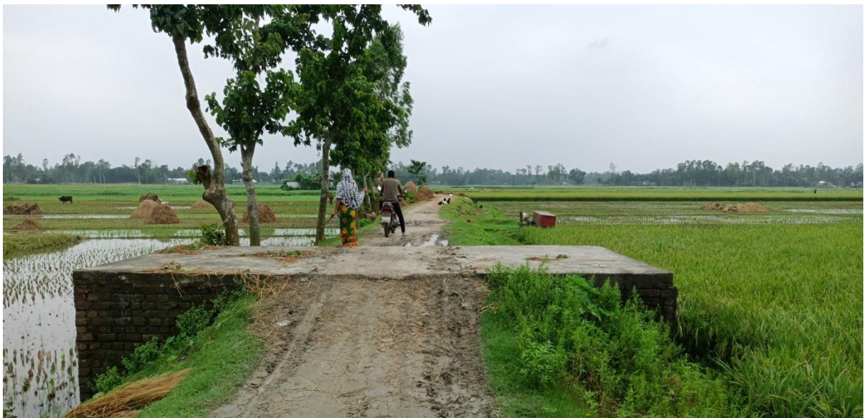
Figure 7: Condition of the visited road alignment at Case Study Union
