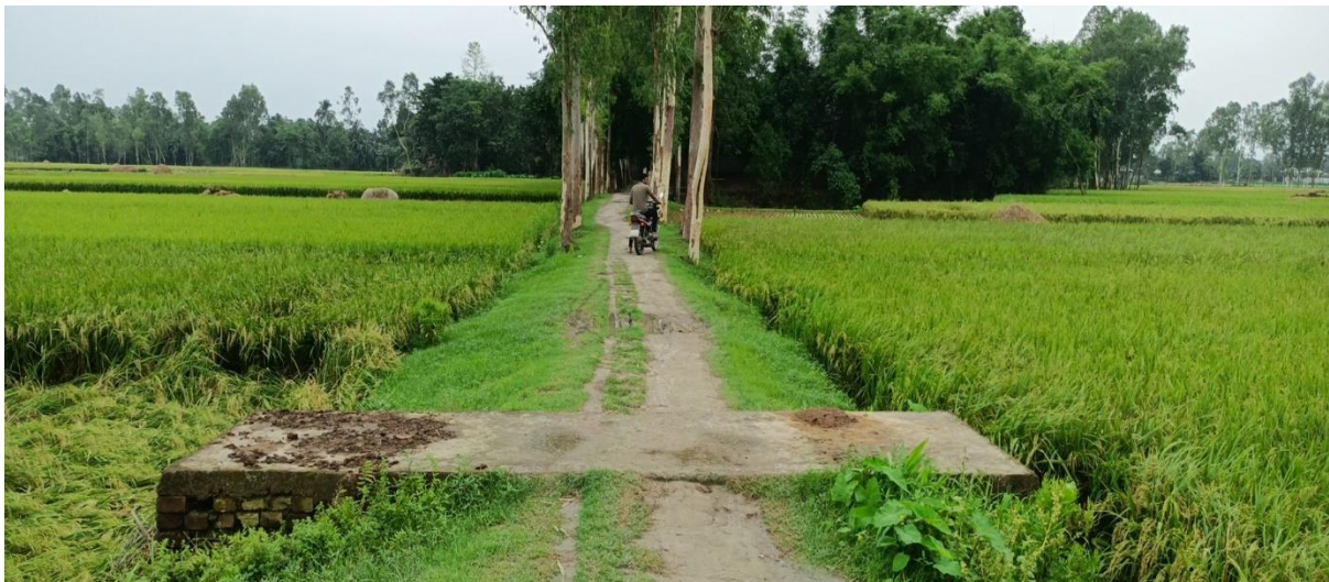
Figure 10: Condition of the visited road alignment at Case Study Union
