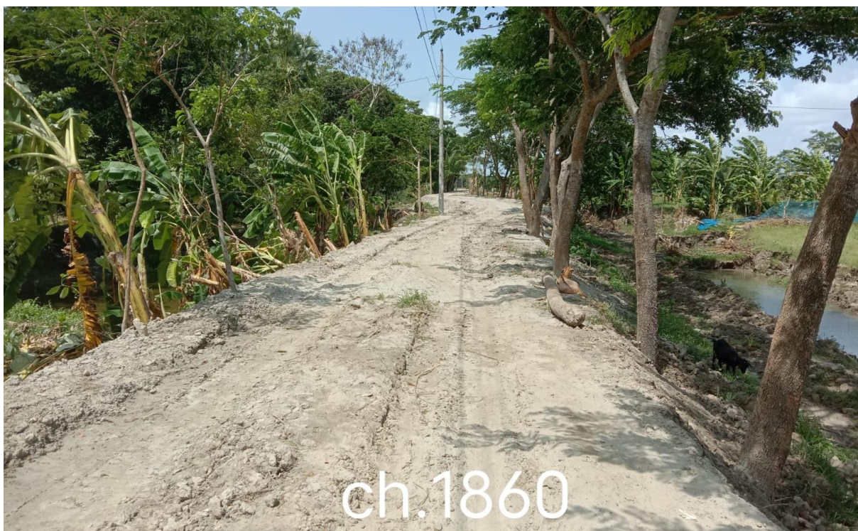
Figure 7: Condition of the visited road alignment at Case Study union
