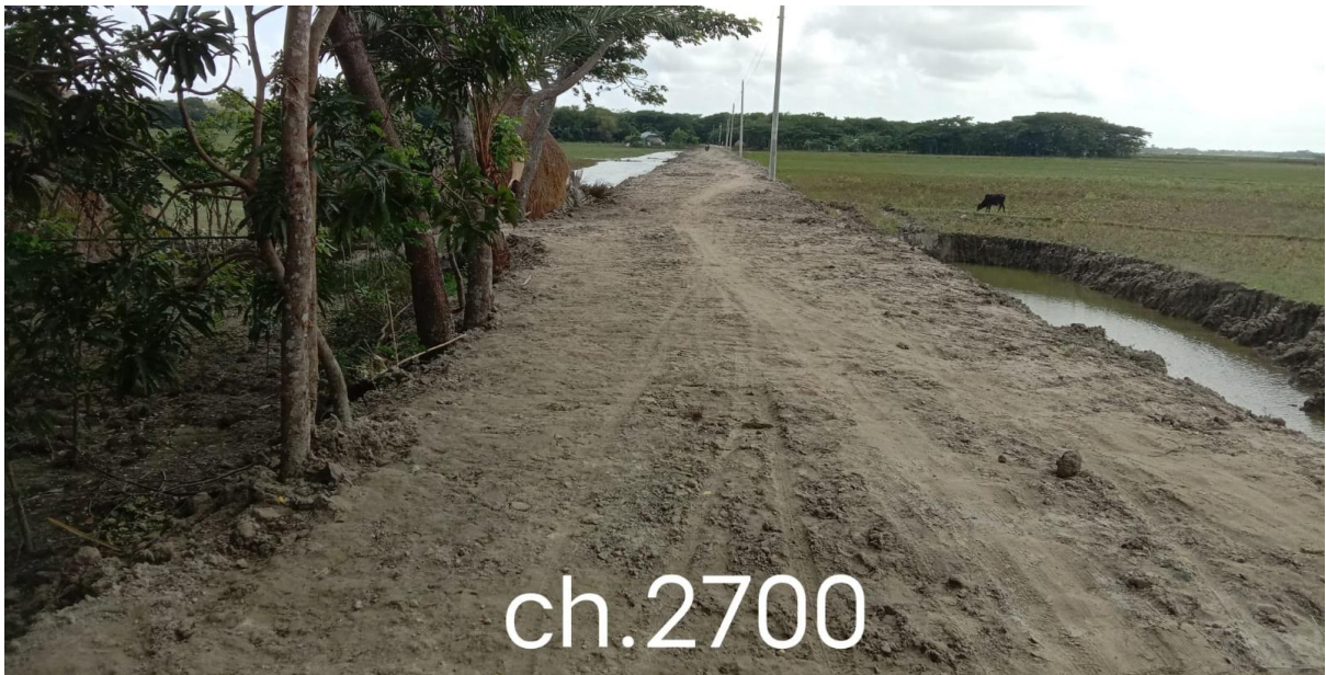
Figure 9: Condition of the visited road alignment at Case Study union
