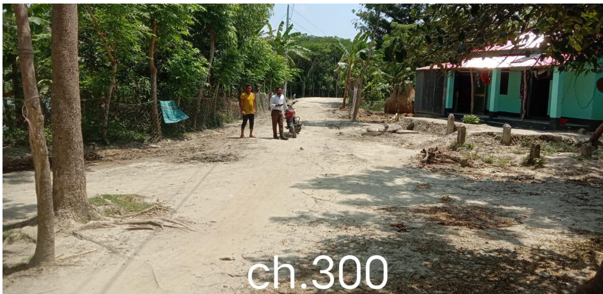
Figure 4: Condition of the visited road alignment at Case Study union
