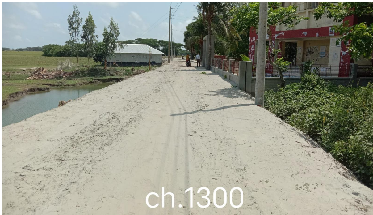
Figure 6: Condition of the visited road alignment at Case Study union
