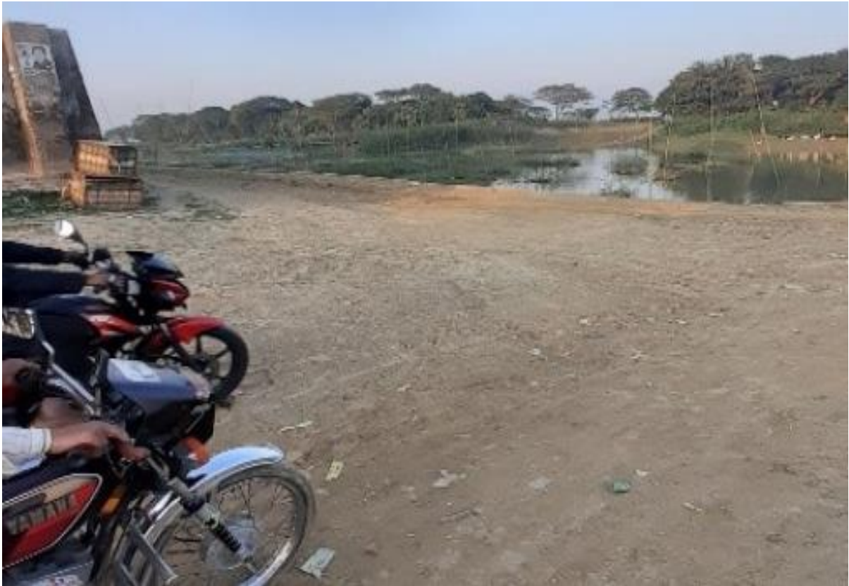
Figure 5: Condition of the visited road alignment at Case Study Union
