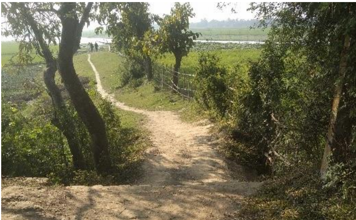
Figure 9: Condition of the visited road alignment at Case Study union
