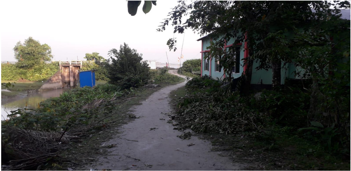
Figure 5: Condition of the visited road alignment at case study union
