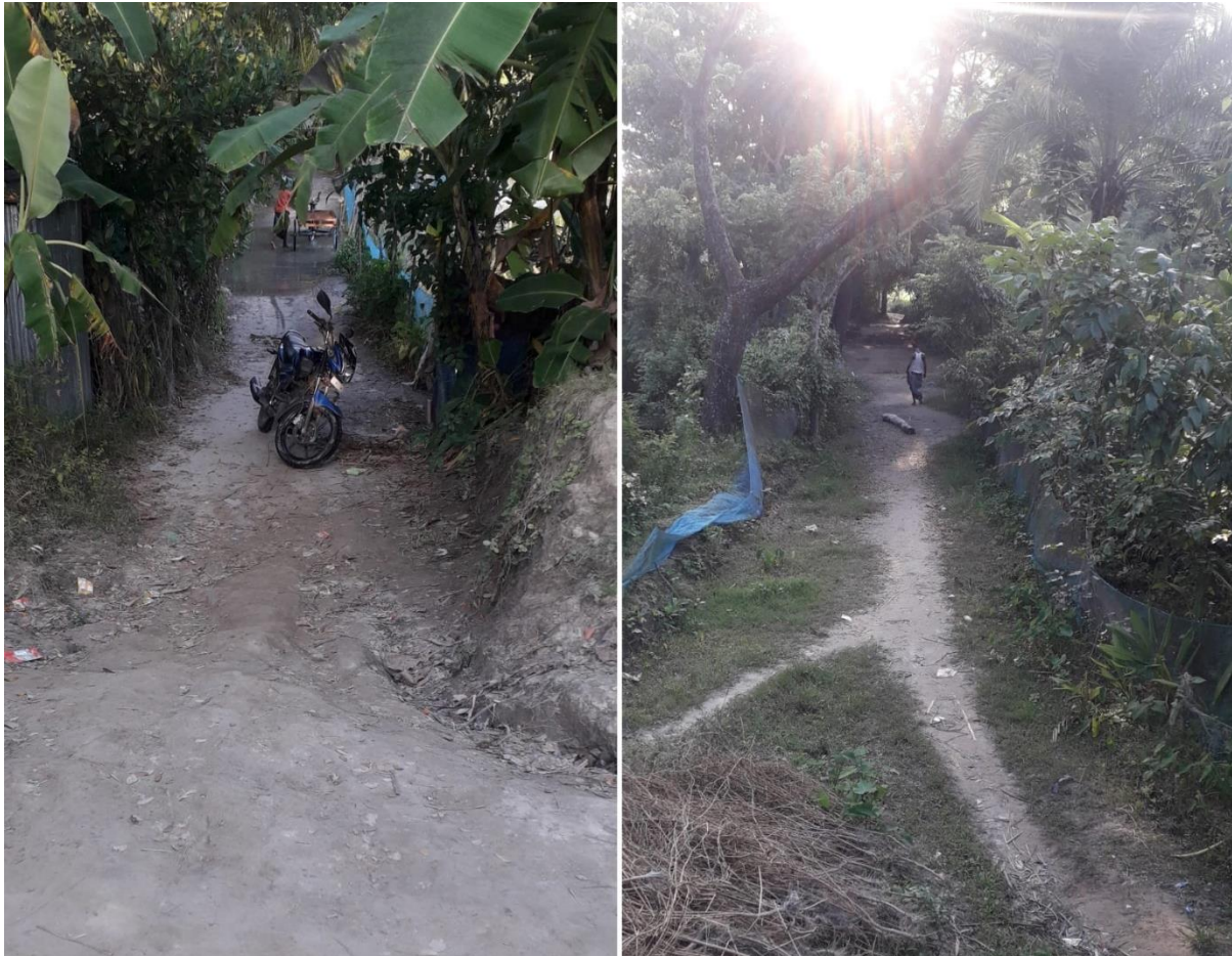
Figure 4: Condition of the visited road alignment at case study union
