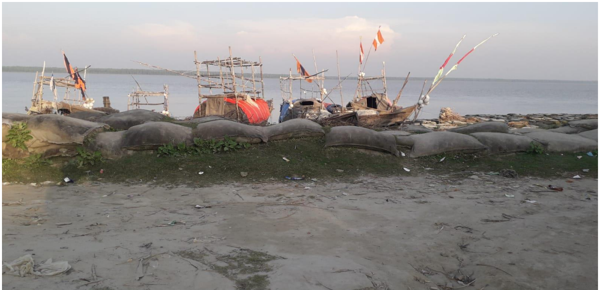
Figure 6: Condition of the visited road alignment at case study union
