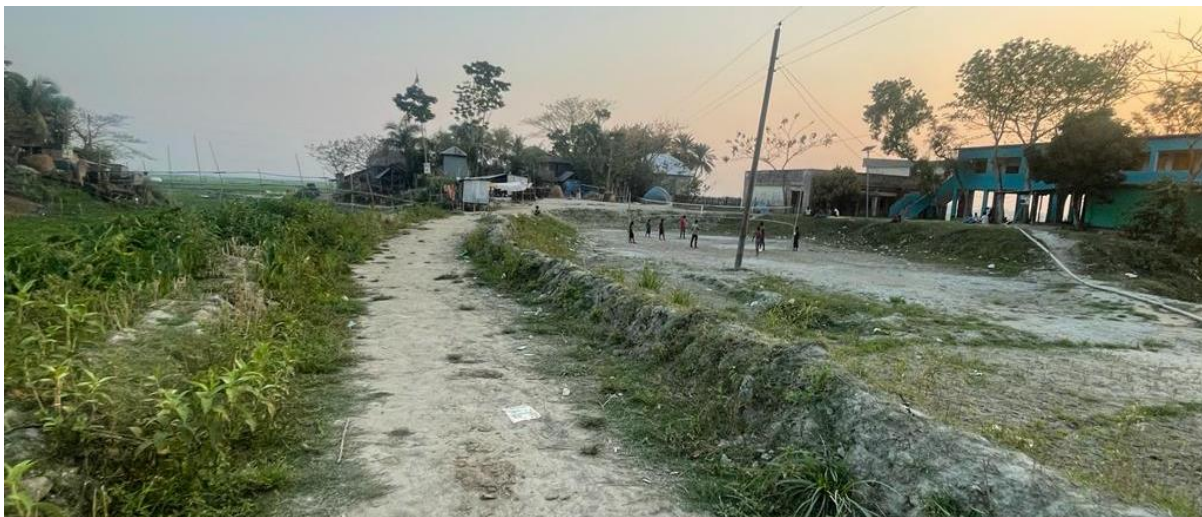
Figure 5: Condition of the visited road alignment at case study Union
