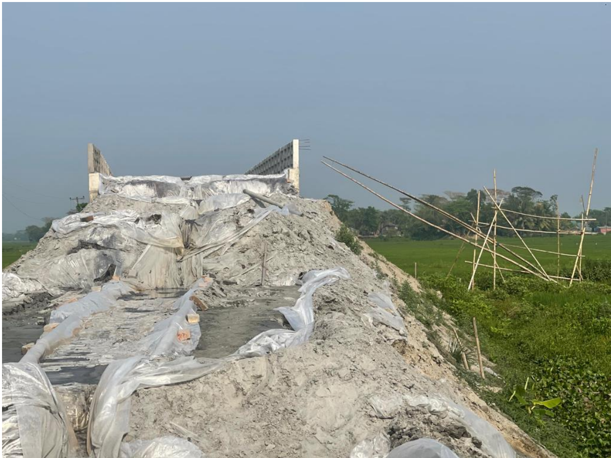
Figure 7: Condition of the visited road alignment at case study Union
