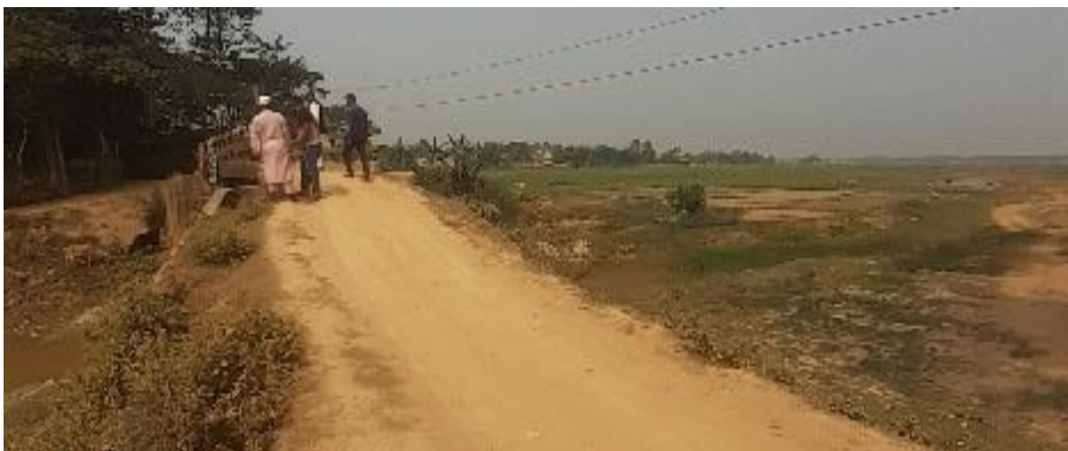
Figure 8: Condition of the visited road alignment at case study Union
