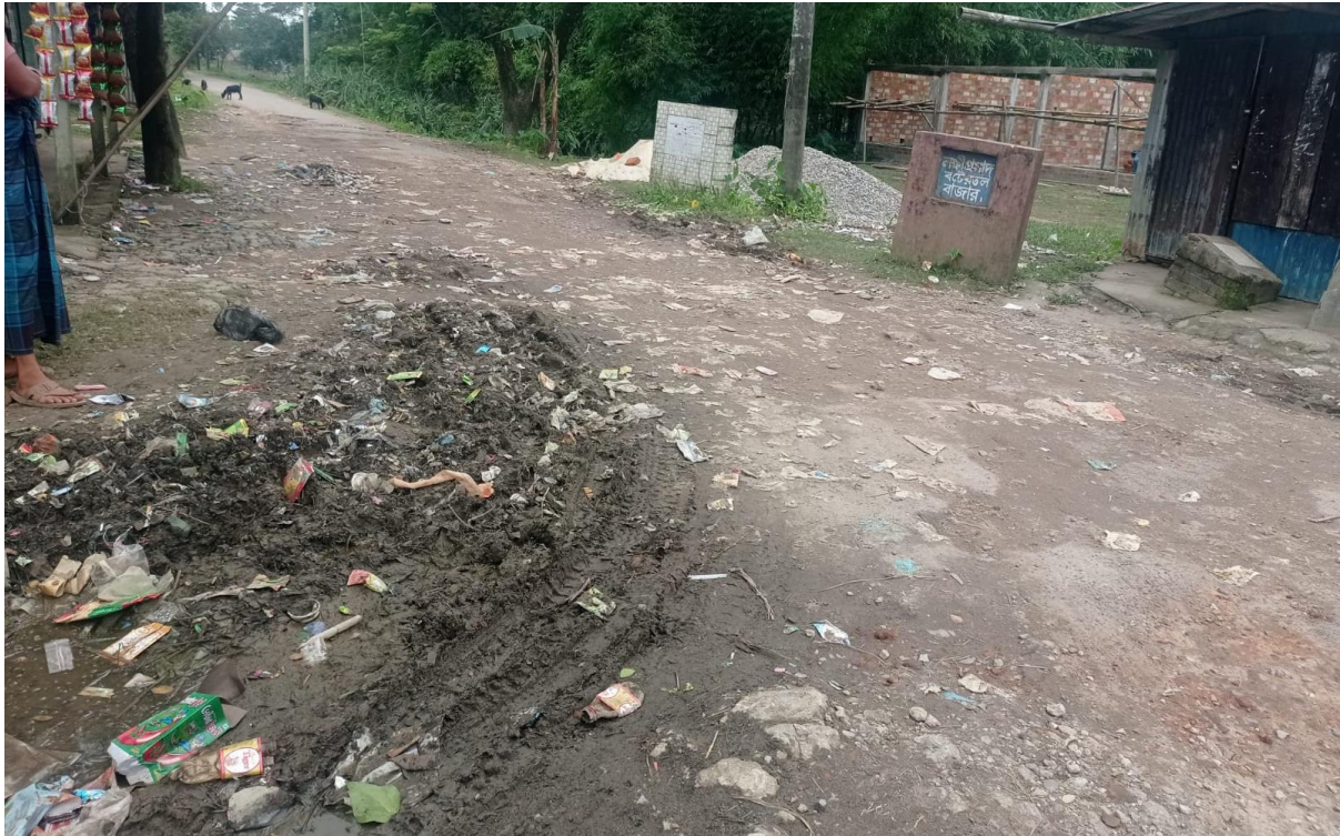
Figure 8: Condition of the visited road alignment at Case Study Union
