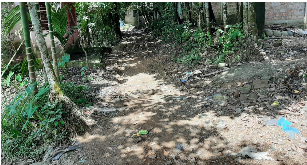
Figure 9: Condition of the visited road alignment at Case Study Union
