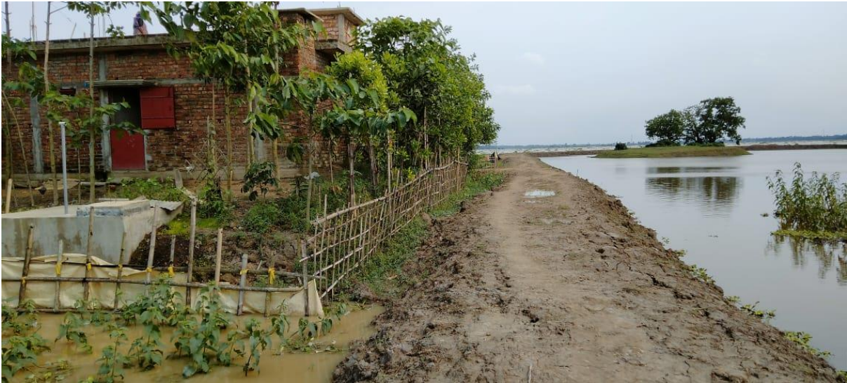
Figure 9: Condition of the visited road alignment at Case Study union
