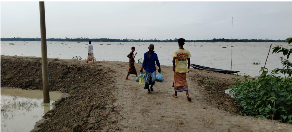
Figure 11: Condition of the visited road alignment at Case Study union
