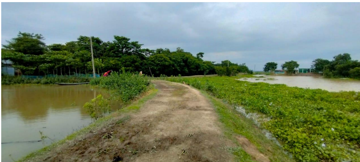
Figure 8: Condition of the visited road alignment at Case Study union
