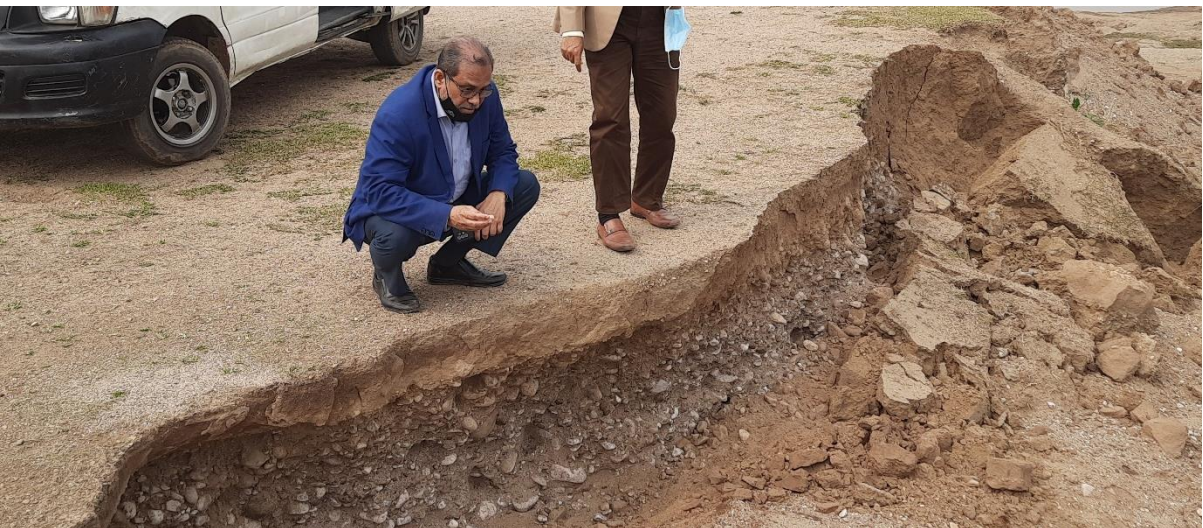
Figure 11: The land sliding due to illegal stone collection
