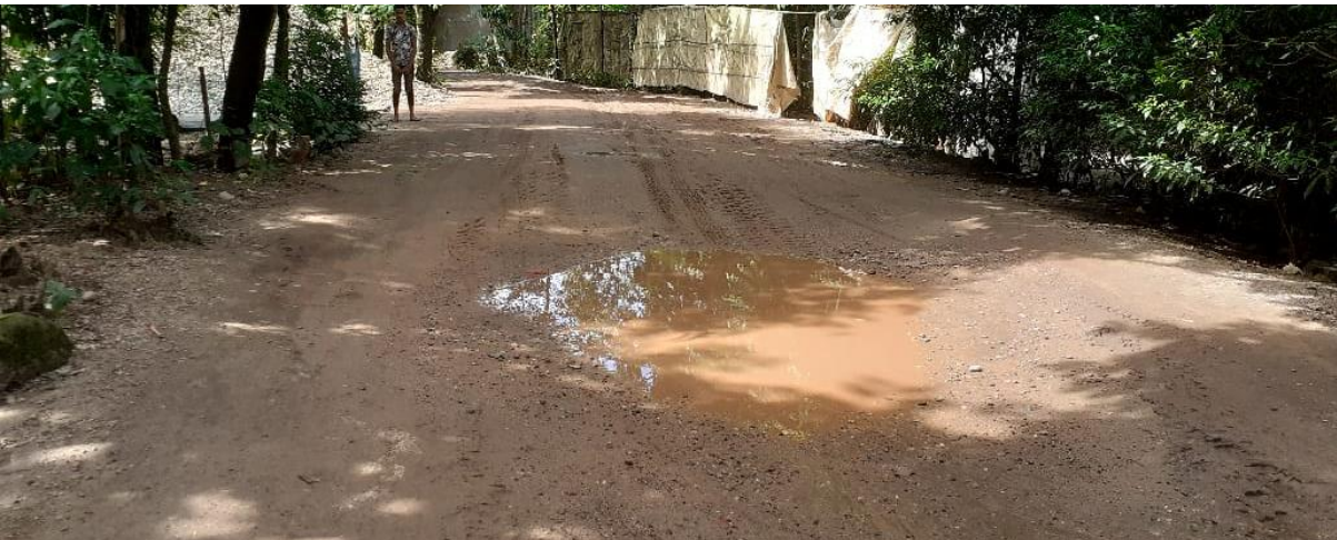
Figure 10: Condition of the visited road alignment at Case Study Union
