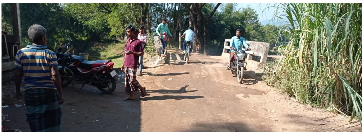
Figure 8: Condition of the visited road alignment at Case Study Union
