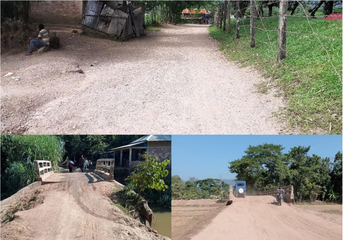
Figure 9: Condition of the visited road alignment at Case Study Union
