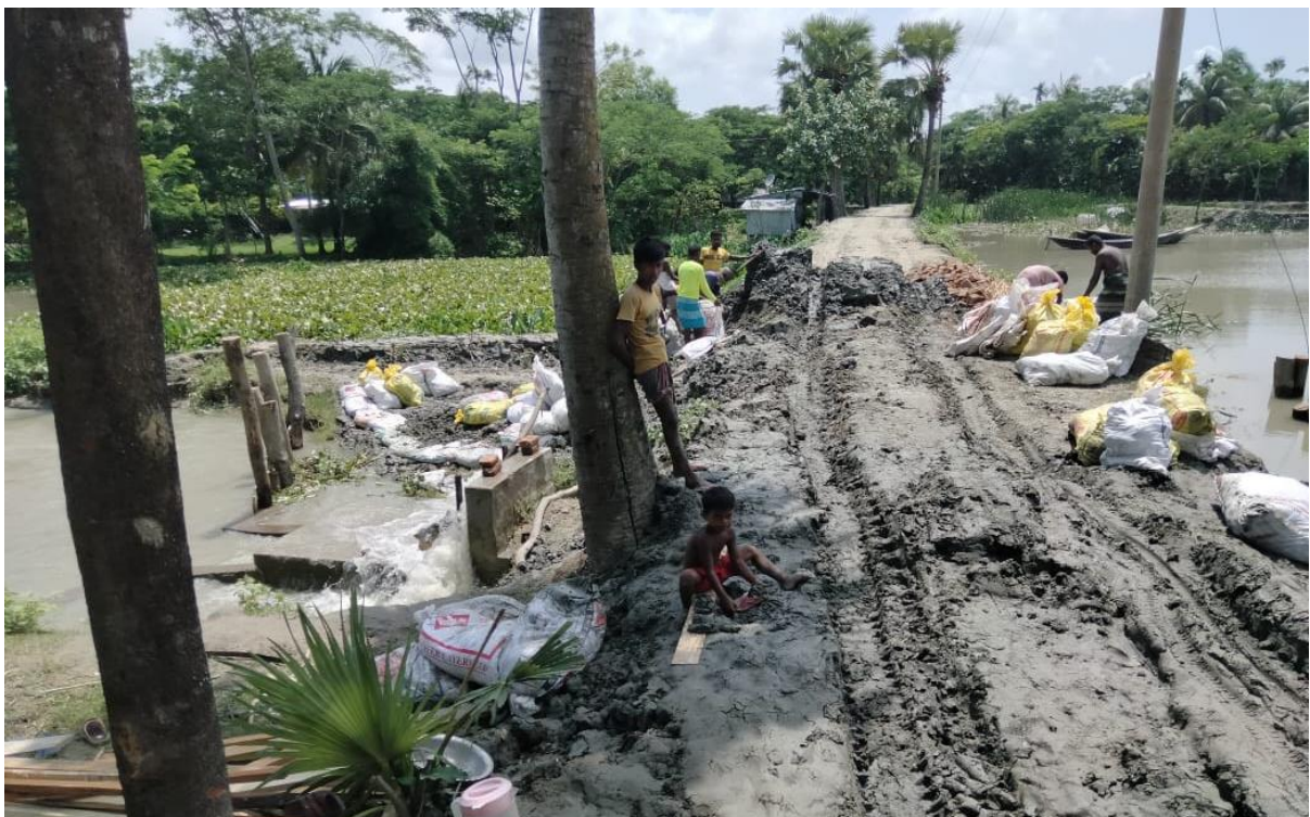
Figure 7: Condition of the visited road alignment at Case Study Union
