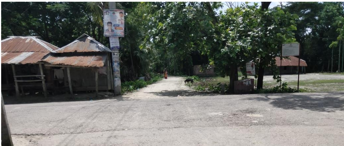
Figure 4: Condition of the visited road alignment at Case Study Union
