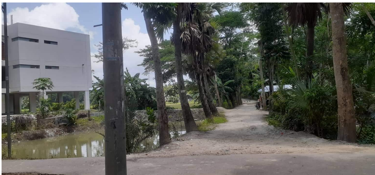
Figure 10: Condition of the visited road alignment at Case Study Union
