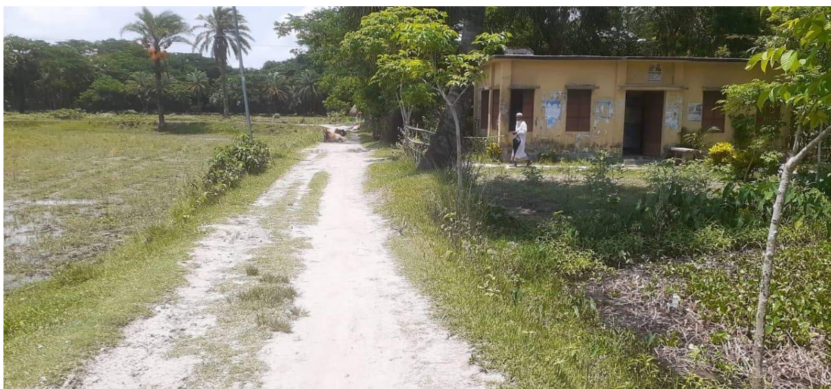
Figure 11: Condition of the visited road alignment at Case Study Union
