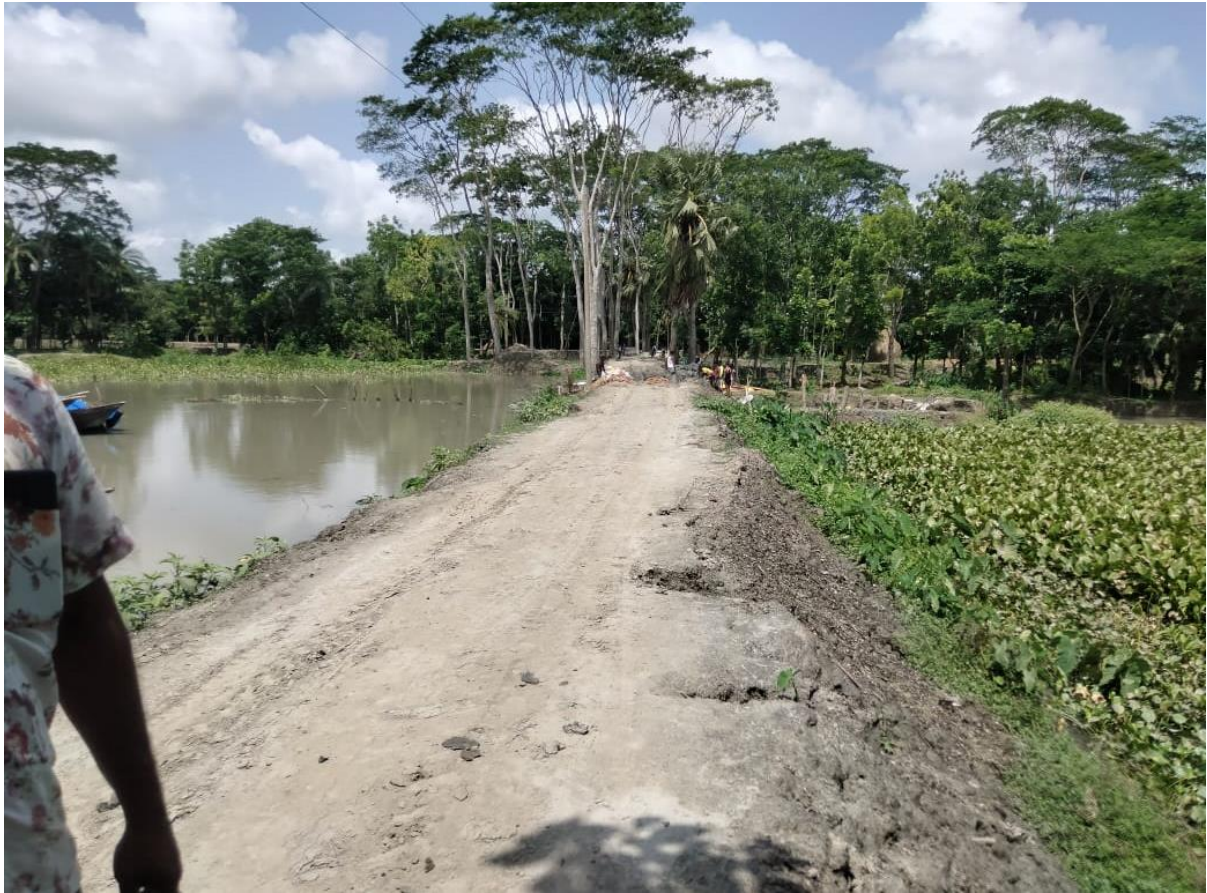
Figure 6: Condition of the visited road alignment at Case Study Union
