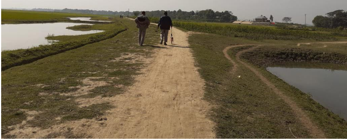
Figure 12: Condition of the visited road alignment at Case Study union
