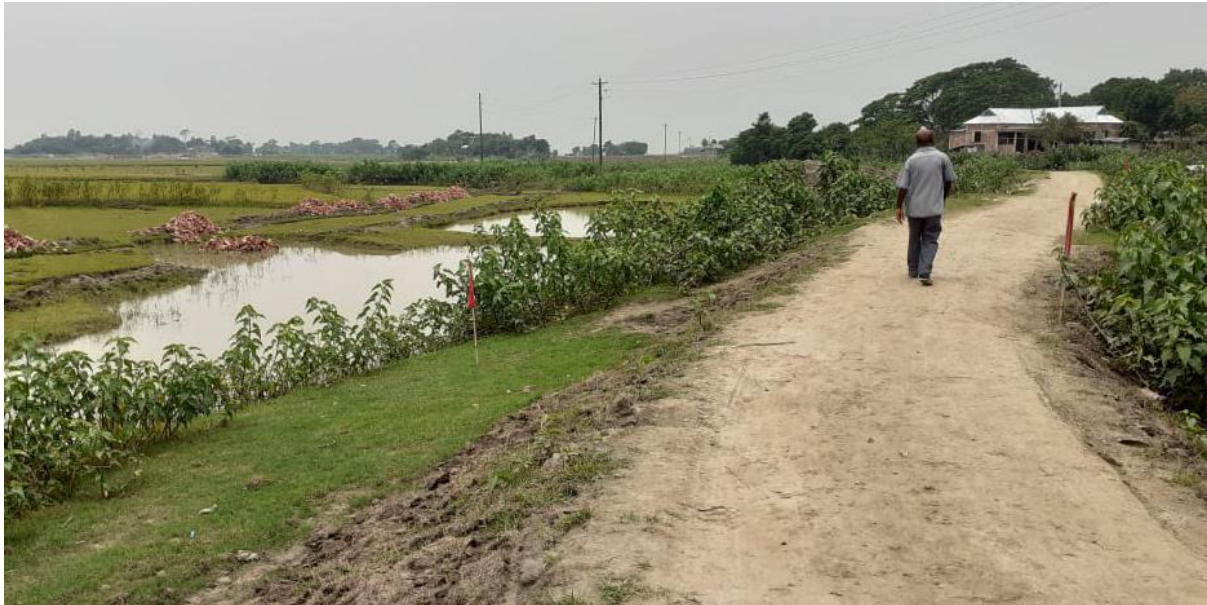
Figure 9: Condition of the visited road alignment at Case Study union
