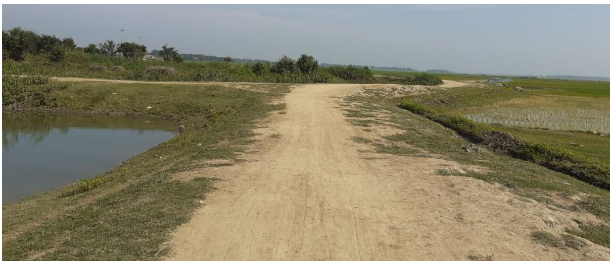
Figure 11: Condition of the visited road alignment at Case Study union
