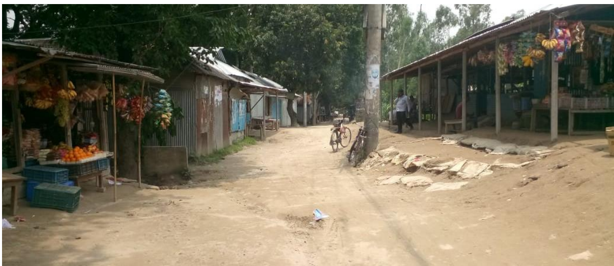
Figure 10: Condition of the visited road alignment at Case Study Union
