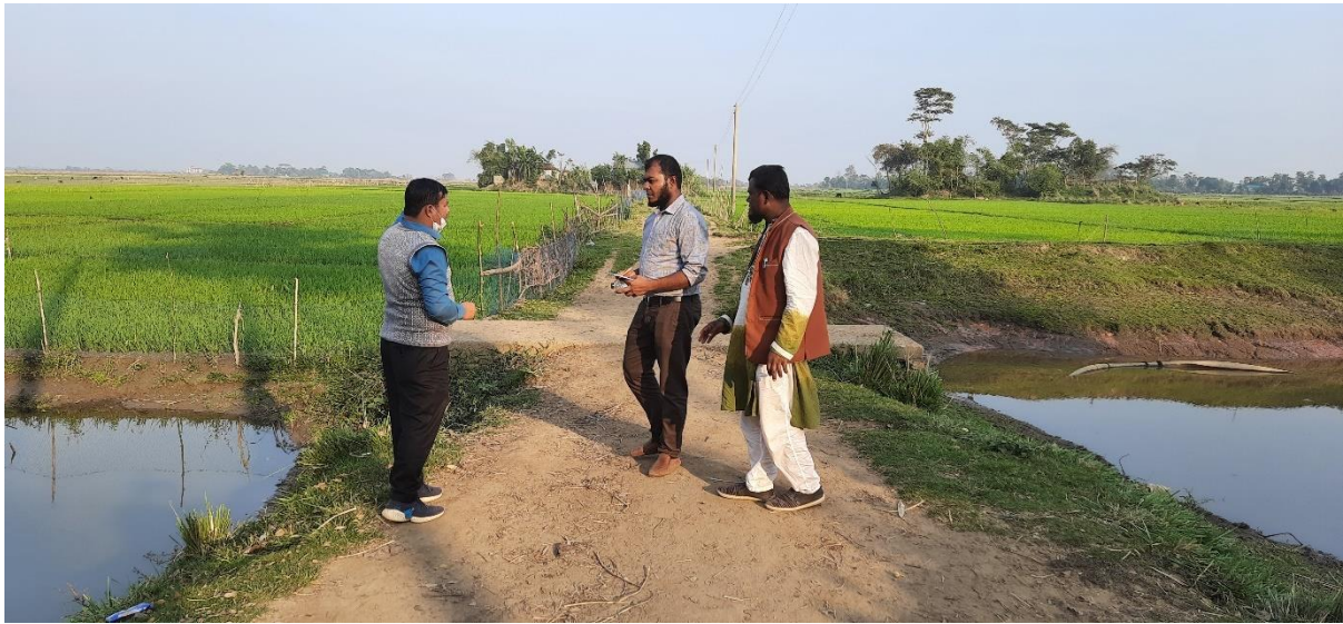
Figure 9: Condition of the visited road alignment at Case Study Union
