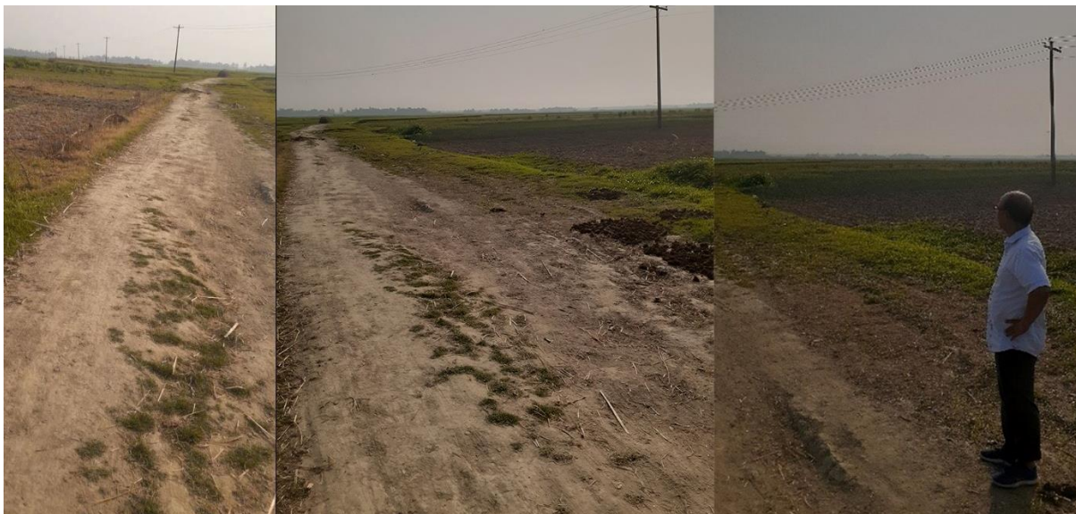
Figure 5: Condition of the visited road alignment at Muksudpur Union
