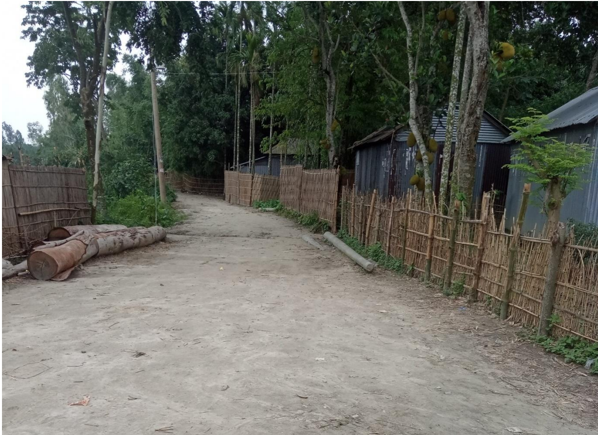
Figure 4: Condition of the visited road alignment at Case Study Union
