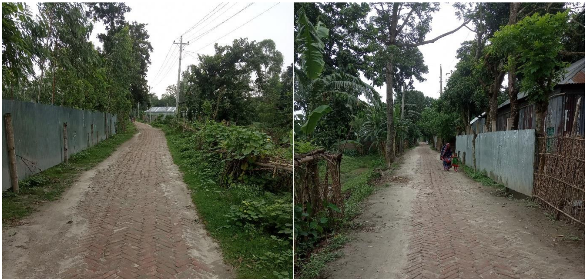
Figure 6: Condition of the visited road alignment at Case Study Union
