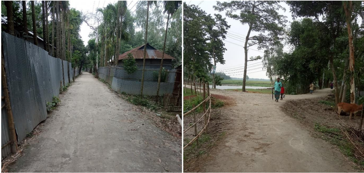
Figure 5: Condition of the visited road alignment at Case Study Union
