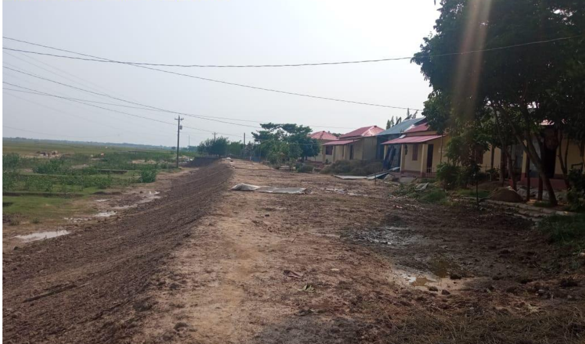
Figure 9: Condition of the visited road alignment at Case Study union
