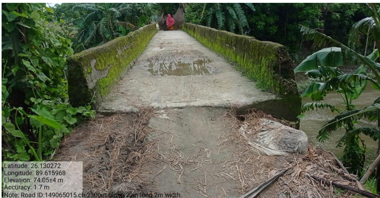
Figure 8: Condition of the visited road alignment at Case Study Union
