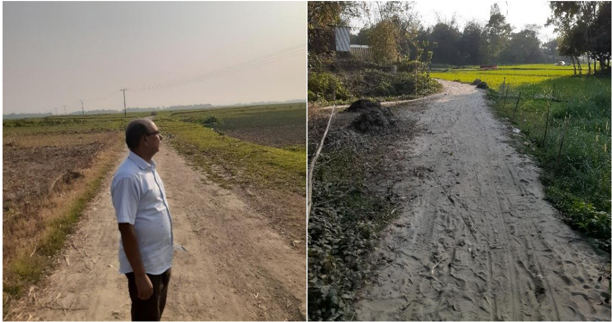
Figure 5: Condition of the visited road alignment at Case Study Union
