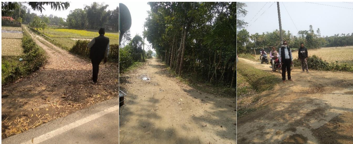
Figure 8: Condition of the visited road alignment at case study Union
