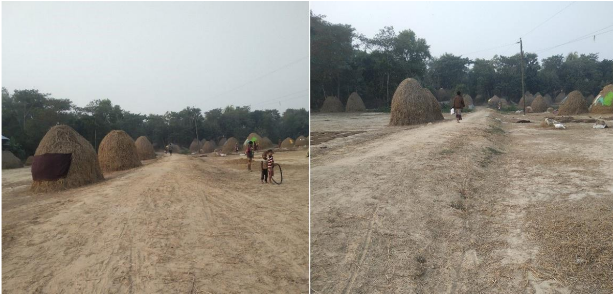
Figure 8: Condition of the visited road alignment at Azmiriganj Union
