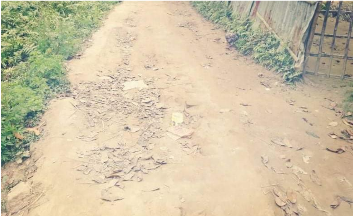
Figure 8: Condition of the visited road alignment at case study union
