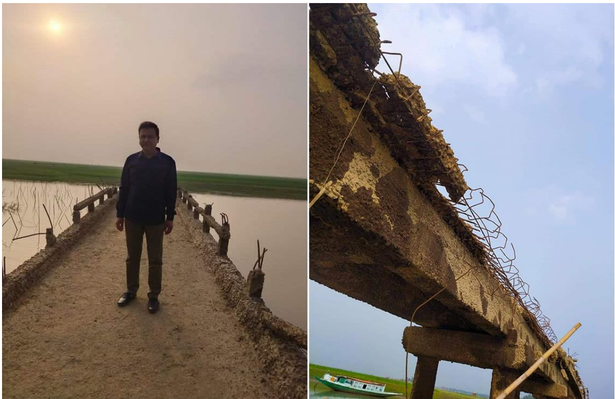
Figure 9: Condition of the visited road alignment at case study union
