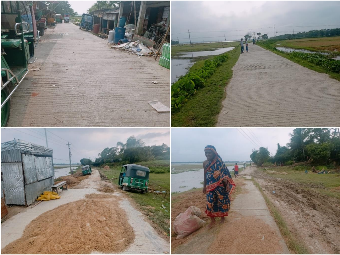
Figure 8: Condition of the visited road alignment (paved part, 690933010)
