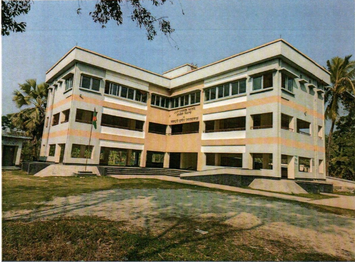
12No Chor Jahanpur GPS CUM DISASTER SHELTER
