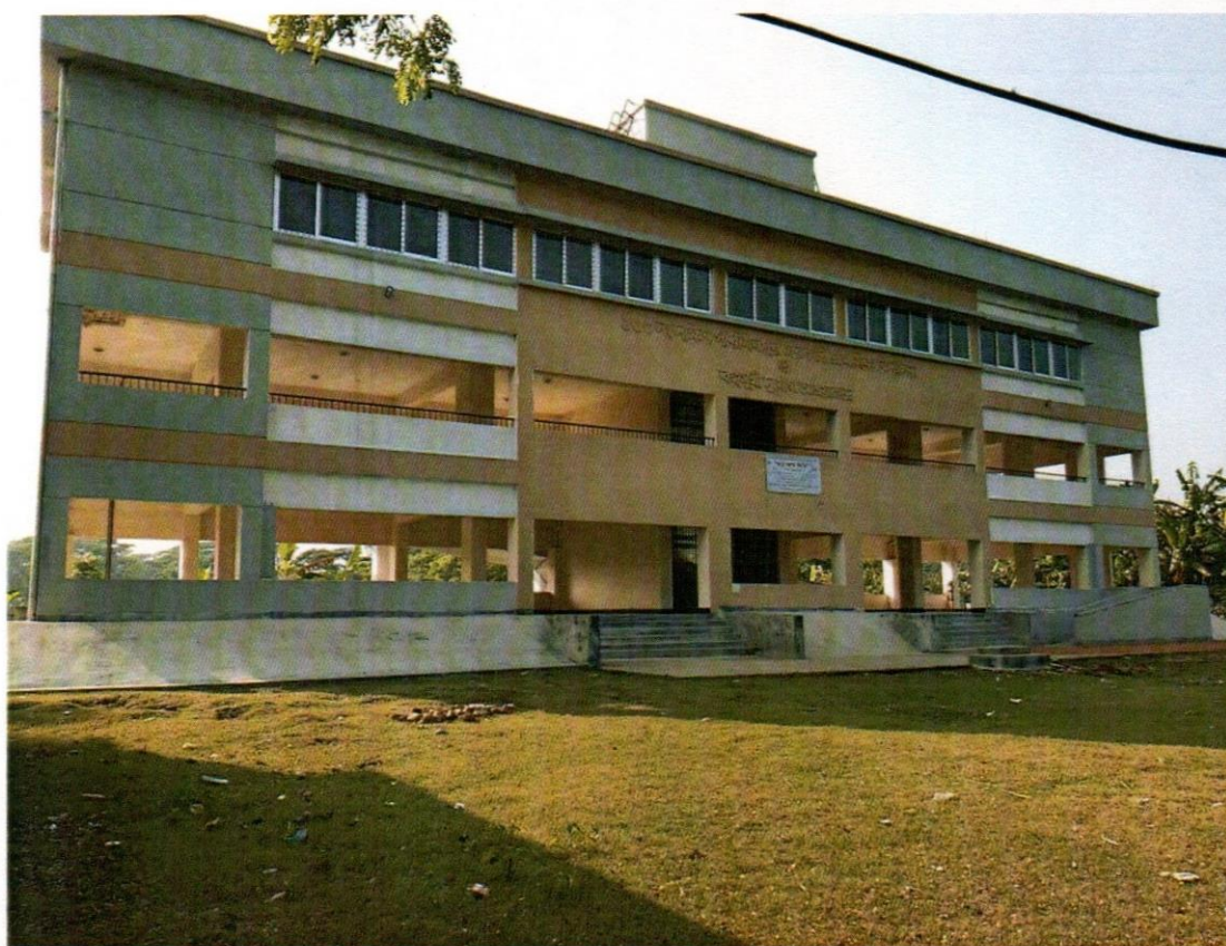
133No South Parshipur GPS CUM DISASTER SHELTER
