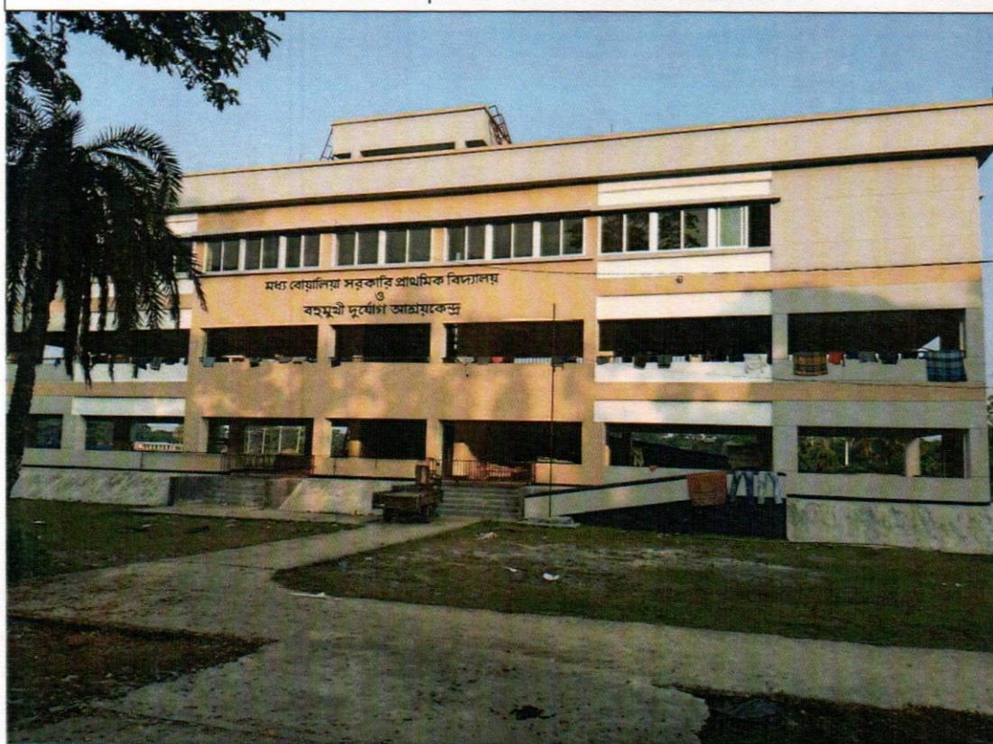
Mid Boalia GPS CUM DISASTER SHELTER
