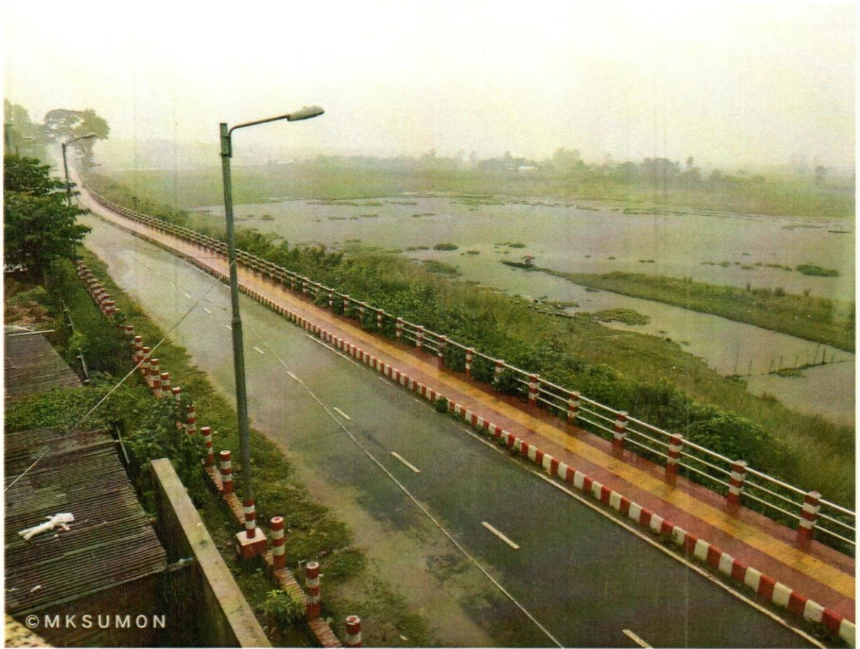
Construction of Fouzdari More to Ferighat Road and footpath @ Jamalpur Pourashava
