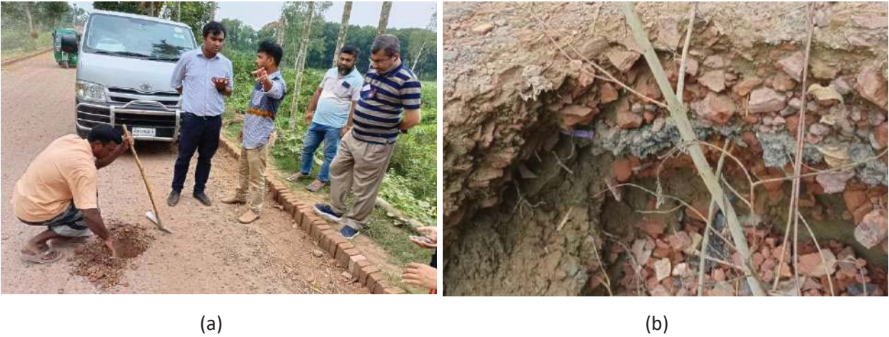
Figure 2: (a) Sample aggregate collection from widened road sub-base. (b) Typical section of widened road (up to sub-base)
