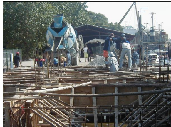
Traditional timber formwork
