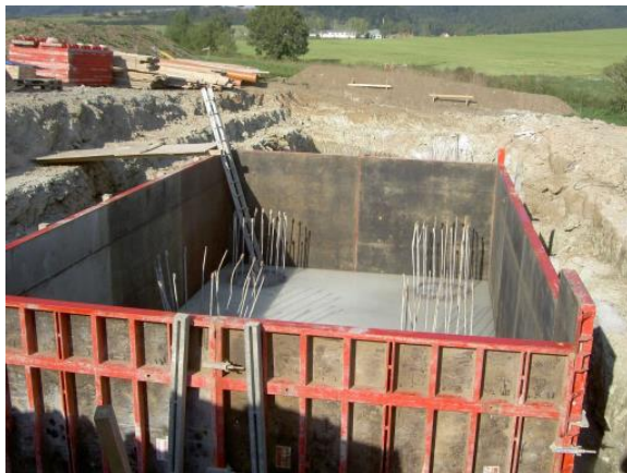
Modular steel frame formwork for a foundation
