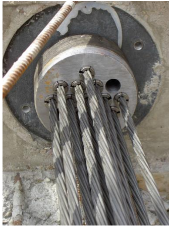
Post-tensioned anchorage
