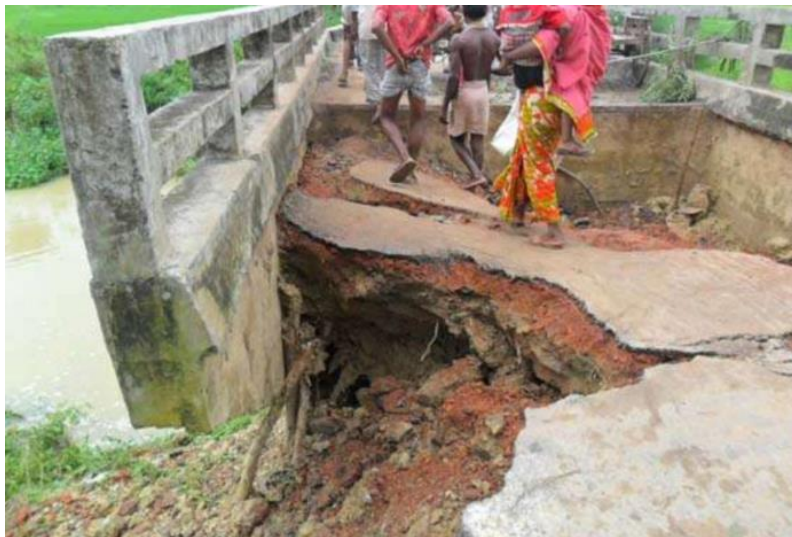
Scour and washout graphic definition and evolution
