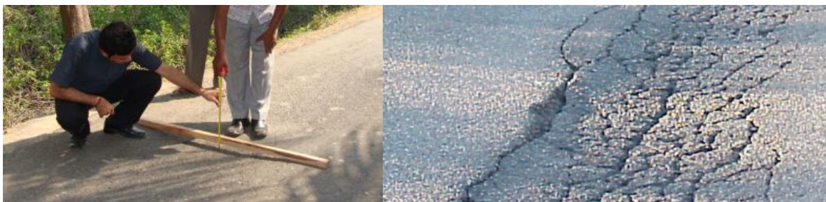
Left: Plastic deformation of the asphalt layer. Centre: Simple depression without rutting. Right: Pathology formation process
