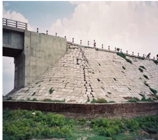
Bridge Failure: Scour at Abutment
