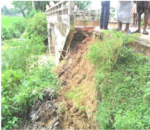
Bridge Failure: Scour at Pier
