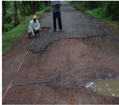
Road Failures: Revelling
