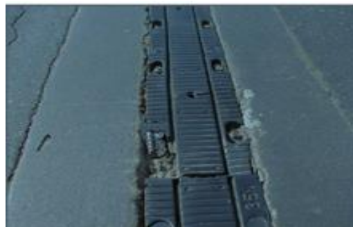
Bridge Failure: Mechanical Devices (Expansion Joints)
