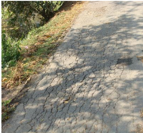
Road Failures: Edge Failure
