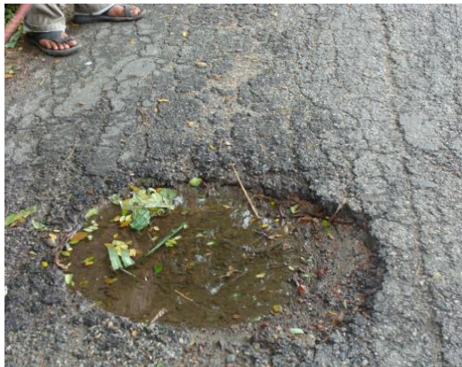
Road Failures: Pothole
