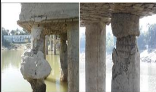
Bridge Failure: Cracks and Spalling
