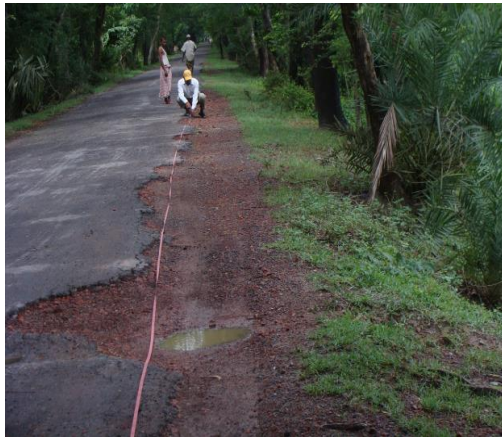
Road Failures: Pothole
