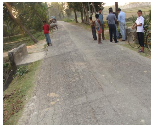
Road Failures: Revelling
