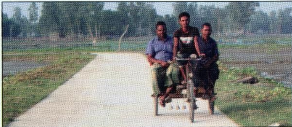
Newly constructed submersible road
