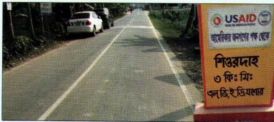
Newly rehabilitated road
